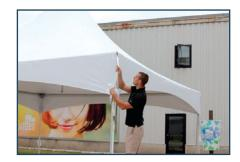
Connect the top carabiner on the outguy strap to the metal loop on the tent bracket.
