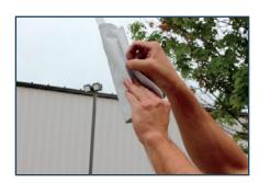
Once the tent is secured to all water barrels, fold the extra out guy strap length into the white vinyl covers with Velcro closure.
